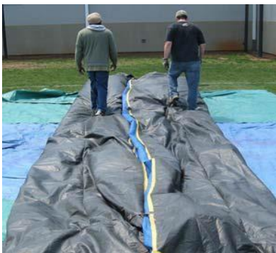
Step 4: After folding the Inflatable twice lengthwise, walk out air towards Ports (Blower tubes).
